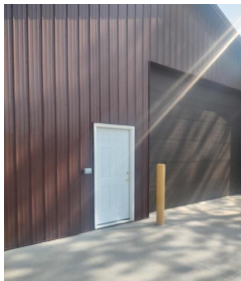
Corey Swanson and his dad moved the man door on the new barn to the front. When it was on the side, it was under rain drip. Much better here.
