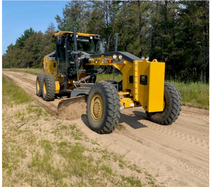
We rented a grader for two weeks to repair the trail. Several members manned the beast.
