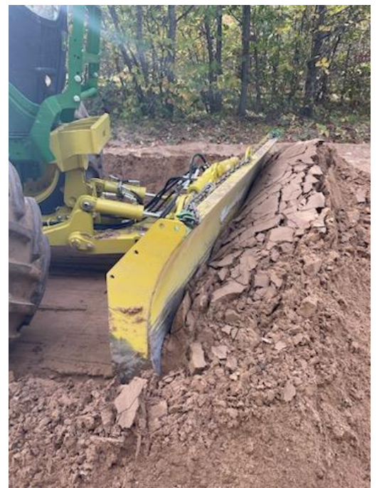
Dan Whitie spent days cutting down the corners on trails. The berms were caused by ORV use in the summer. IF we don't cut them down now, they will be HUGE in snow season.
