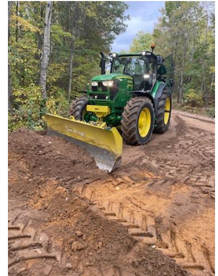
Dan works to cut down the big berms on the corners.
