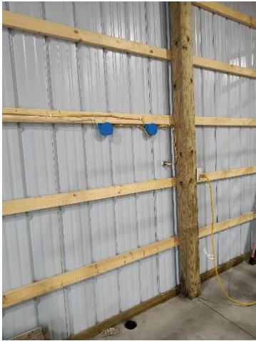
Greg mounted electrical boxes on the walls and on the ceiling for lights.
