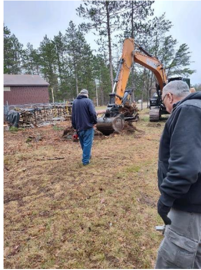
Pat was busy locating wires and unhooking propane tank.
