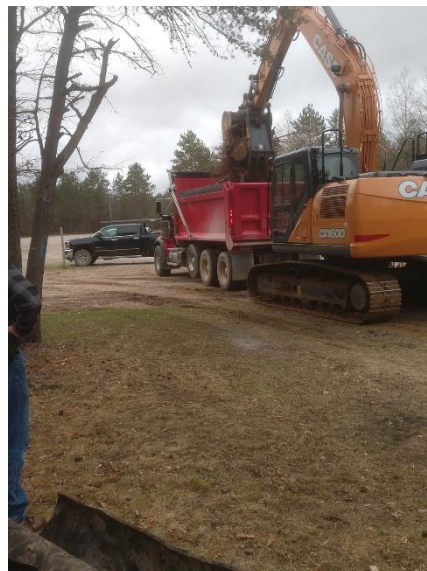
The excavator picked up stumps and loaded into the truck.
