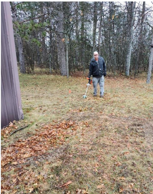
Pat had to locate the underground wiring before the excavator could remove stumps.
